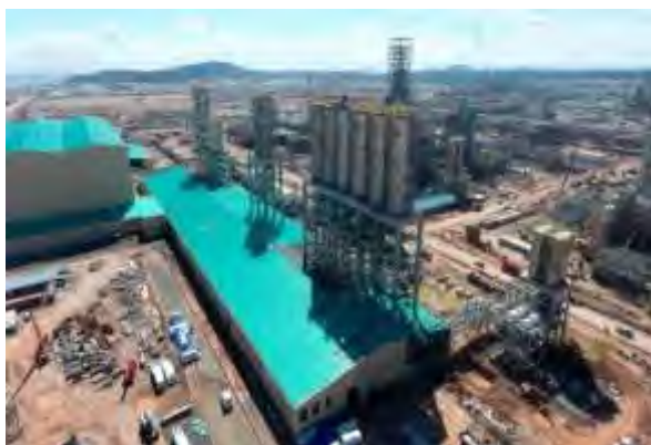
RAPID Package 12A - ASRS Warehouse, Malaysia
