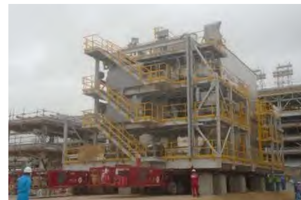
MEI Work for PKG 4 - EPC P2 - U&O Duqm Refinery Project Oman
