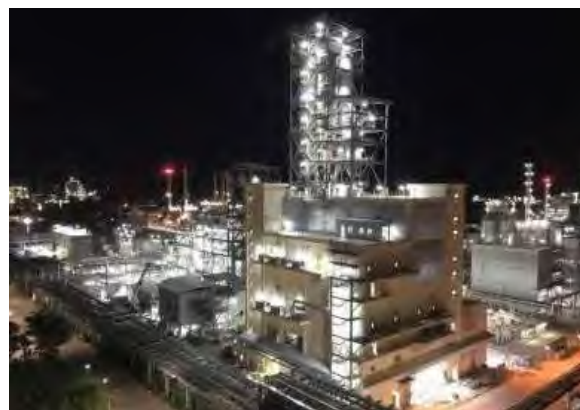
IRPC PPC & PPE Project, Thailand
