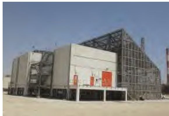
Petrokemya Power Station Project, Saudi Arabia
