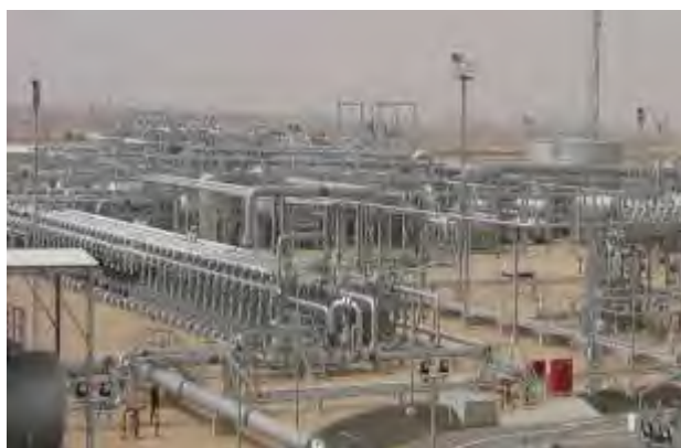
GC32 Gathering Center Project - Electrical & Mechanical Package Kuwait
