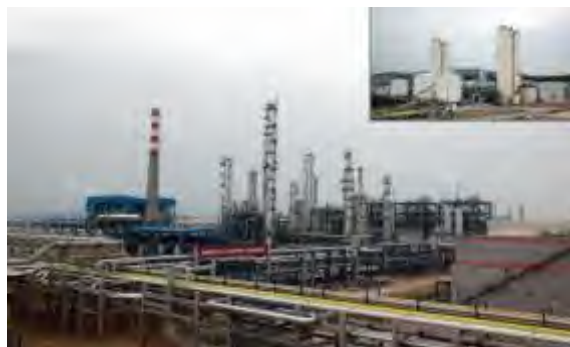
IGCC Project in Fujian Refining & Petrochemical Complex
